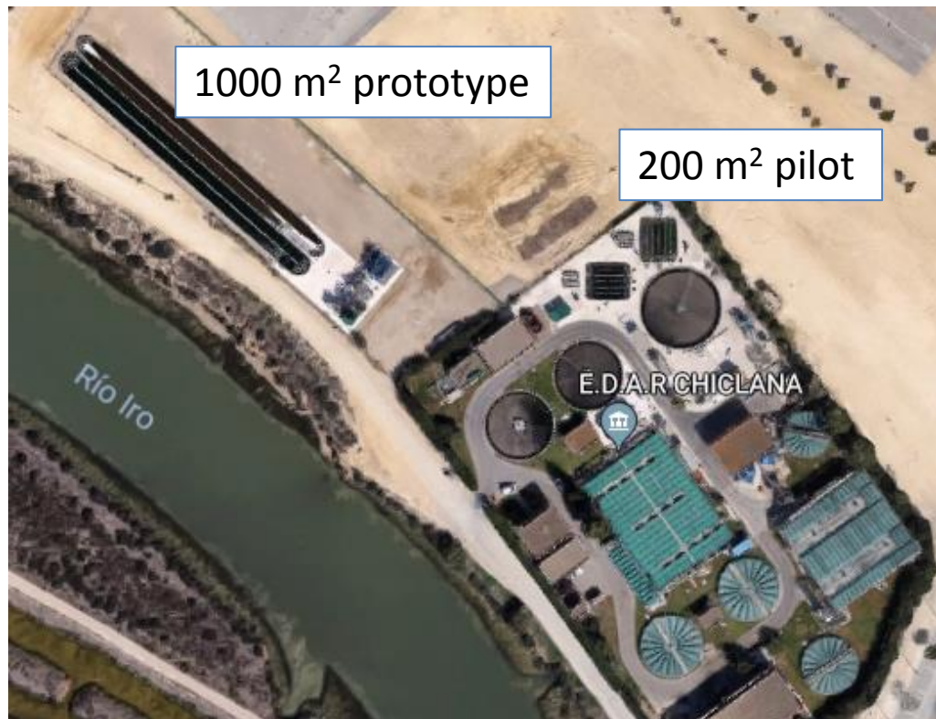
WWTP at Chiclana de la Frontera (Andalusia, Spain)
